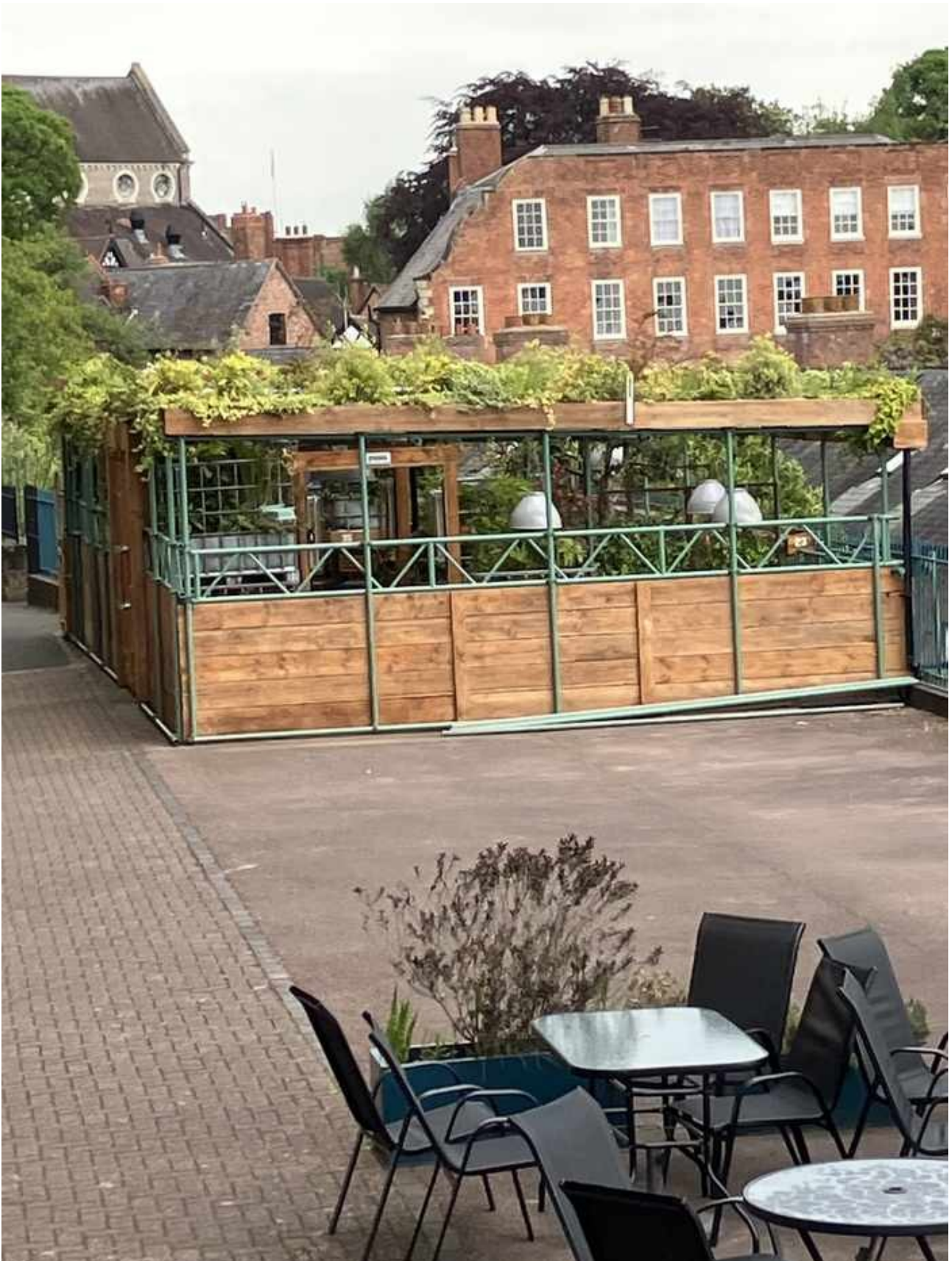
Photograph 3: Ground-level front view showing the solid horizontal timber planking, green metal scaffolding poles, and open metal railings above. The scale of the structure is clearly visible.
